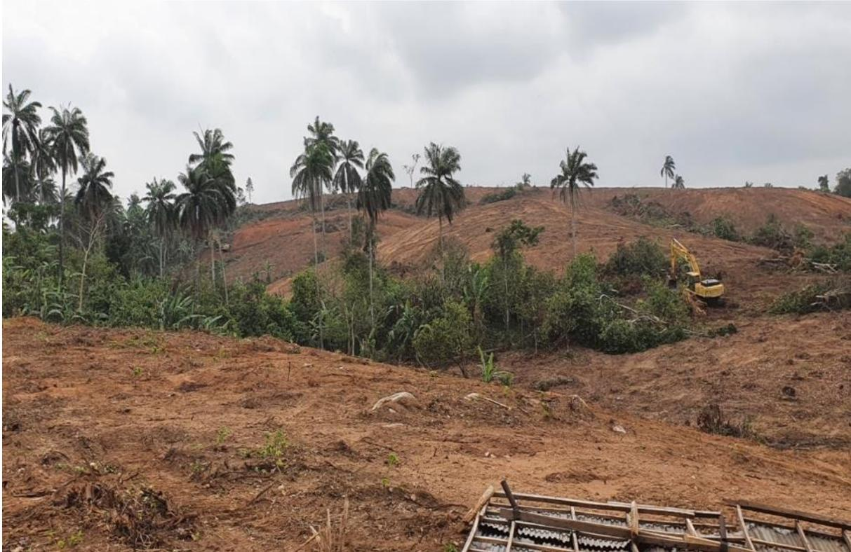
**Figure 16-2. ROM Pad Clearing and Grubbing Activity (17th of March 2021)**
