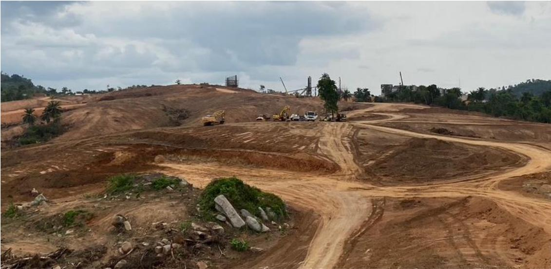
Figure 10-1. Pit surface area being stripped of vegetation and prepped for overburden stripping (9th March 2021)
