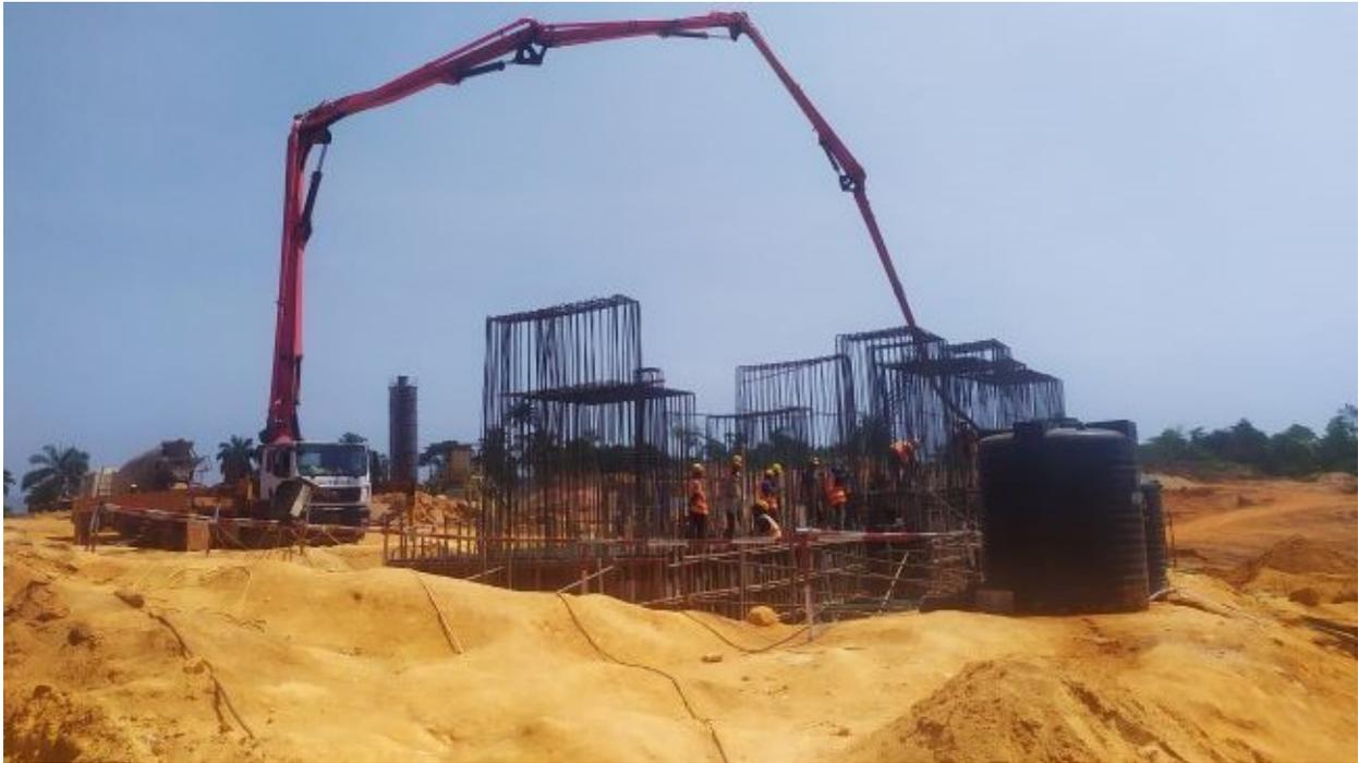
Figure 2: Casting of Ball Mill Foundation
